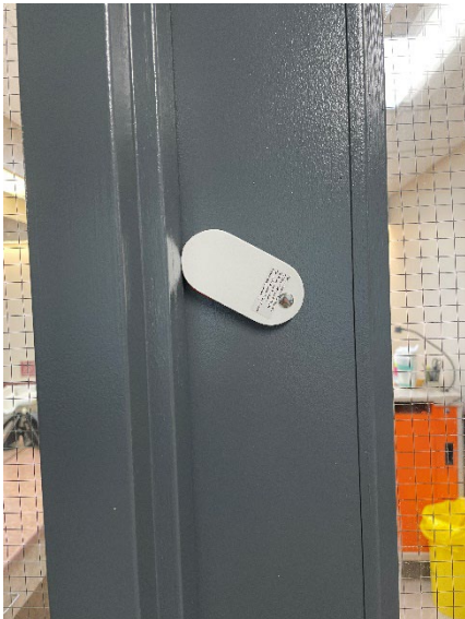
Door flag displaying only white shows that the room has been evacuated and has not been re-entered.
