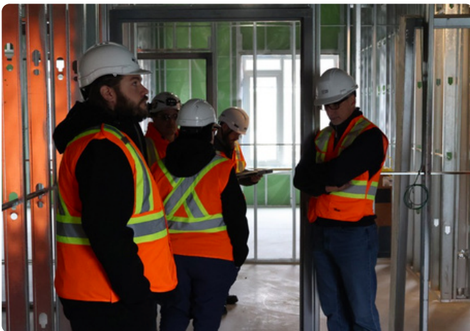
The DRDH Team inspecting a resident space with completed interior framing
