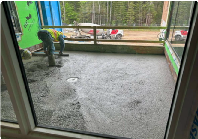
Second floor concrete porch pour and leveling in progress.
