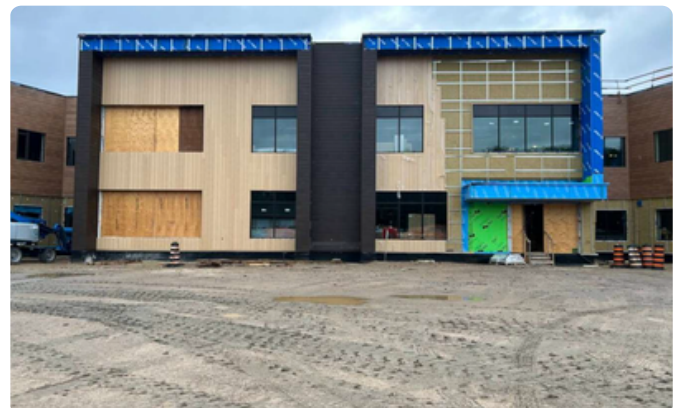
View of the front entrance with cladding install in progress.
