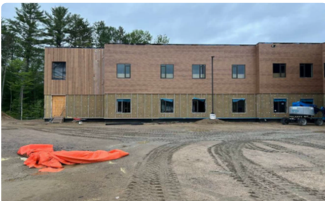
View of a resident room with exterior insulation installed and cladding in progress.
