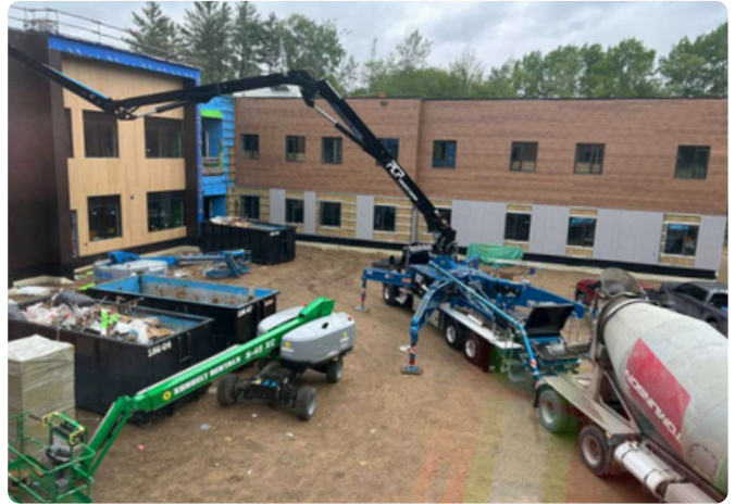
View from second floor towards courtyard, showing concrete trucks pouring porches.
