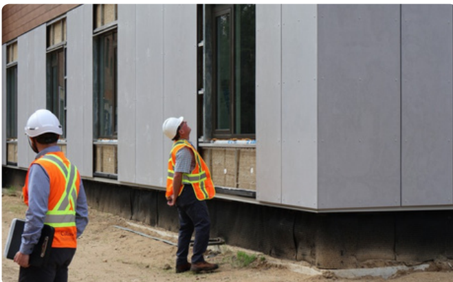
DRDH Board Chair, David Cox, inspecting the newly installed concrete cladding.
