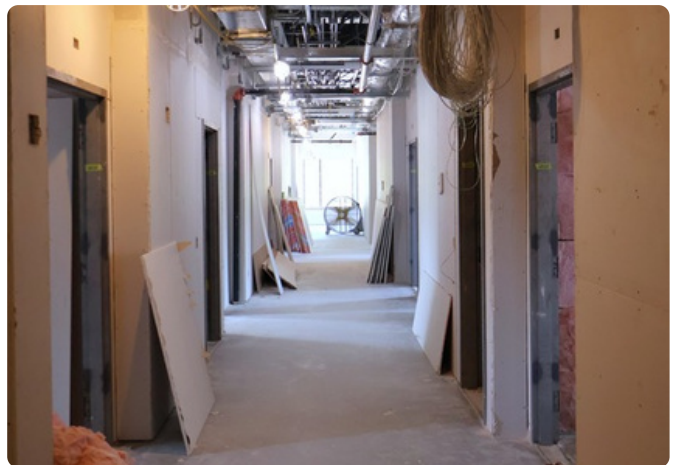
Second floor corridor showing drywall and insulation installation progress.
