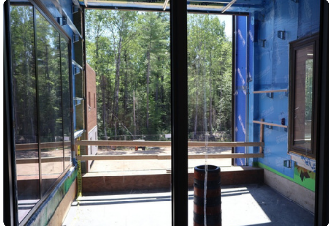
View from a second-floor porch overlooking the adjacent conservancy.
