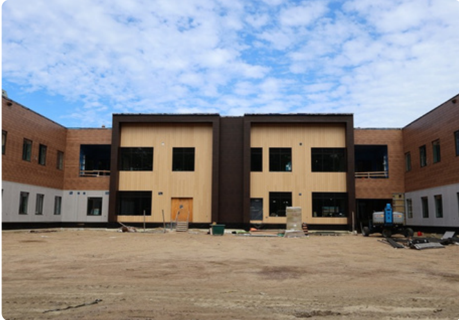
Rear courtyard exterior showing architectural concrete cladding installed along the main floor.
