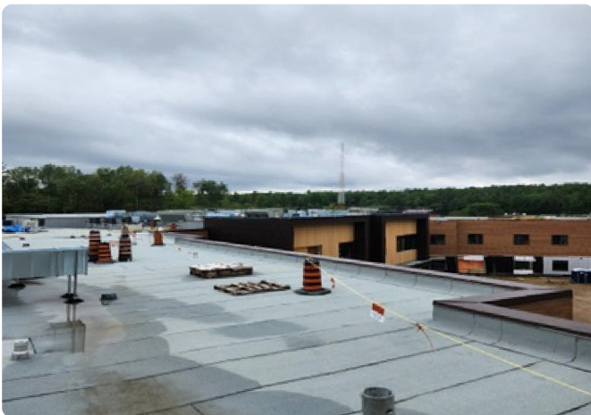
View of the completed roofing membrane near the main entrance.
