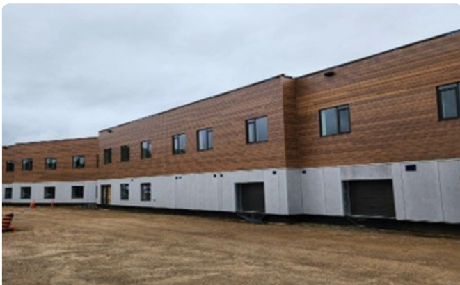
Exterior view of the Shipping and Receiving area, with cladding and panel installation completed.
