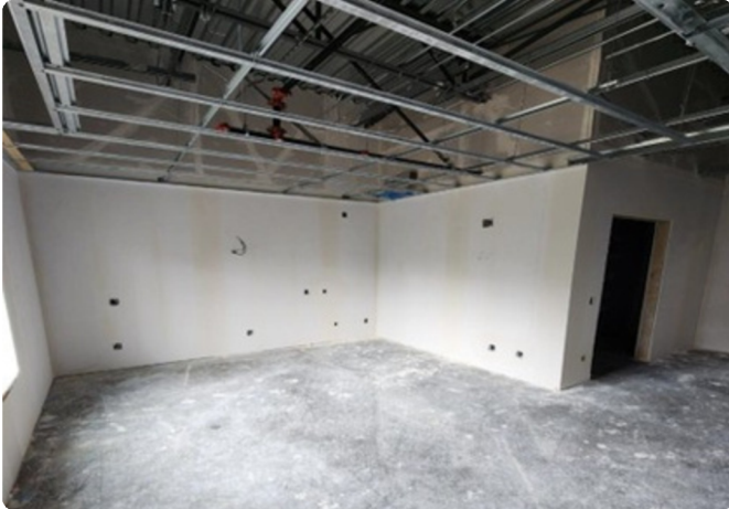
Private room on Level 2, showing progress on drywall installation and the adjoining bathroom.
