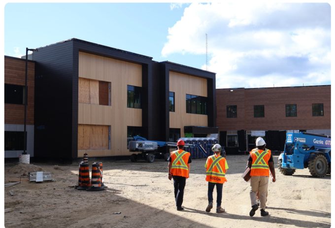
Windows near building entrance will remain boarded to allow materials to pass through.
