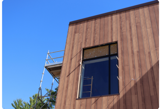
Upper level window installation and finishing is ongoing.
