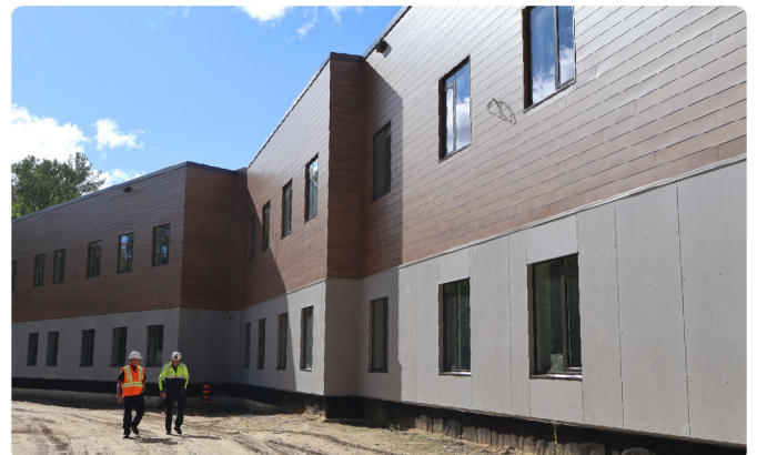
Exterior view of the cladding and panel installation completed.
